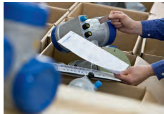
Commissioning of flowmeters
